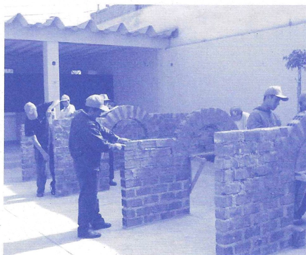
Practical activities of the workshops on gardening and bricklaying.
